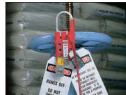
Lockout gate valves
