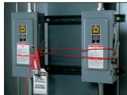
Lockout single or multiple electrical disconnects
